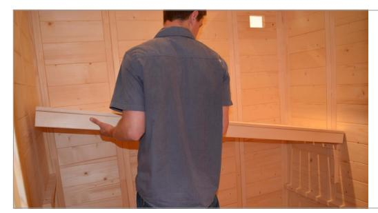
STEP 22 - Place the upper bench onto the upper bench supports. Once the upper bench is in place screw it into the right and left bench supports using (4) 4x60 screws, two on each side and in between the slats. Then, use (4) 4x60 screws and attach the rear of the bench to the rear wall from below the bench. Place one screw into each wall element section by drilling through the rear of the bench.
