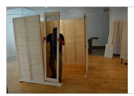
**STEP 12** - Install the narrow glass wall element section with the edge clips facing the door opening.
