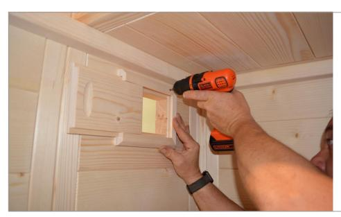
**STEP 28** - Locate the vent cover and position over the wall opening. Attach with (40) 3.5x40 screws.
