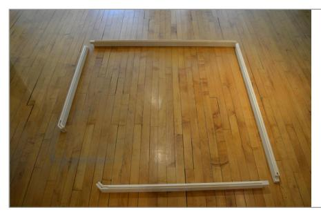
**STEP 1**- Locate the (4) bottom rails and position as shown. Overlap the corner joints and be sure the rails are square to each other. Drill a 1/8" pilot hole in the corner joints and secure rails to each other using a single 5x70 screw in each of 3 corners.
