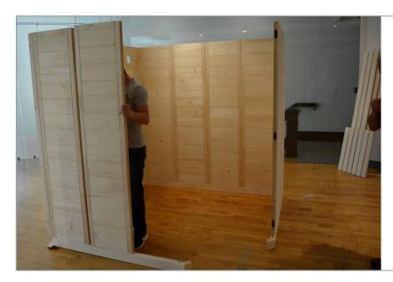
**STEP 11** - Install (1) of the narrow wall elements (N) on the other short wall (this will connect to the wall element you installed in step 3.)
