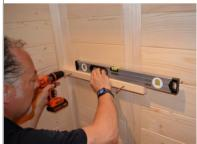
**STEP 19** - You will now install the bench supports. On the shorter left sauna wall and longer right sauna wall of the sauna, from the floor measure 34" and make a pencil mark. Position the top of the 23" upper bench support at the mark and use a level to ensure that the support is level to the ground. Then screw the upper bench support into the wall element sections using 5x70 screws. Do this with both the right and left bench supports.
