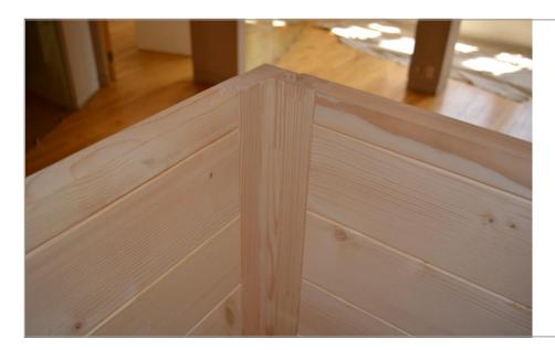
**STEP 4** - Verify that the element wall sections are square to the rails, perpendicular to each other, and that the flat top of the wall elements and corner posts align.
