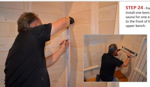
**STEP 24** - For the side bench installation, you need to install one bench support on the front inside wall of the sauna for one end of the bench. The other end will attach to the front of the upper rear bench creating an "L" shaped upper bench.
