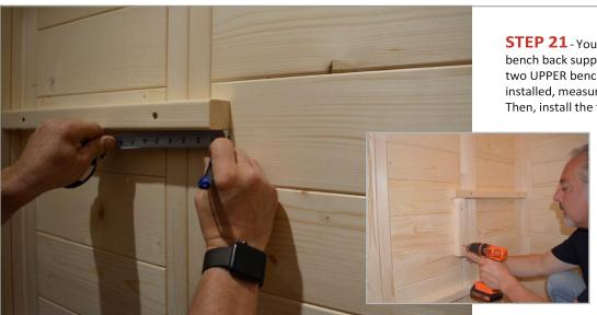
**STEP 21**-You will now install the lower bench back supports. From the front of the two UPPER bench supports that you just installed, measure ¾" back and make a mark. Then, install the two lower backrest supports
