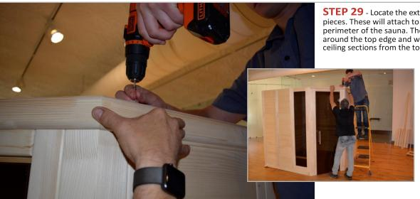
STEP 29 - Locate the exterior ceiling trim pieces. These will attach to the exterior top perimeter of the sauna. The pieces create an "L" around the top edge and will be screwed to the ceiling sections from the top using 3.5x40 screws.
