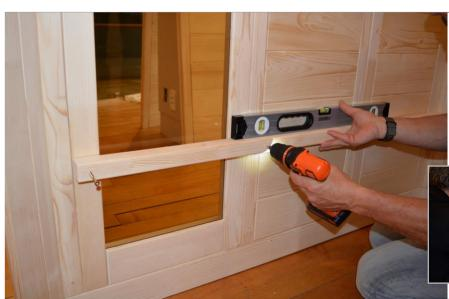
**STEP 20**- For the lower bench supports, repeat step 19 but measure up from the floor 16" and make a mark. Install the right and left longer 52" bench supports, noting that the lower bench support on the shorter left wall will cross the window and be screwed into the window panel.
