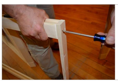
**STEP 15** - Locate the doorframe and remove the bottom board that was used to secure in shipping. SAVE THIS BOTTOM BOARD.
