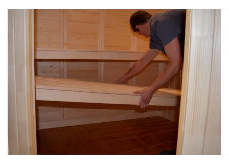
**STEP 23** - Place the lower bench on the lower bench supports. Since the lower bench is intended to slide in and out (it can be used as a step or as a full bench) it is not to be screwed into place.
