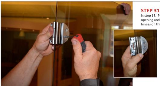
**STEP 31** - Find the board you set aside in step 15. Please it on the floor of the door opening and the place the glass door with hinges on this board. (This allows you to install
