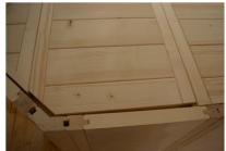
step 18 - From the top of the sauna lay the (3) ceiling element sections in place. The side to face "up" is indicated, and the placement of the sections is intuitive. It is not necessary to screw the ceiling sections to the supports. A proper sauna needs airflow and should not be airtight. However, if your ceiling sections are not laying flat and if you can see gaps of light between the roof sections and the ceiling supports you can screw them down as desired to tighten the fit.
